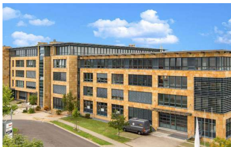
SCAT headquarters near Frankfurt Airport: development, production and logistics in one complex.
